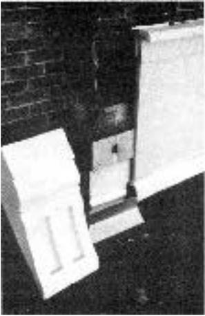
**Figure 1.** To duplicate a missing piece of ornament, a sheet-metal contractor formed galvanized metal on a brake. Inverted dentils are soldered to the back of the body.
