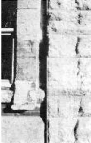
Figure 4. Simulated "marble" blocks around windows were made by covering existing concrete with a patching compound, scoring the compound to look like mortar joints, and sprinkling with marble dust.
