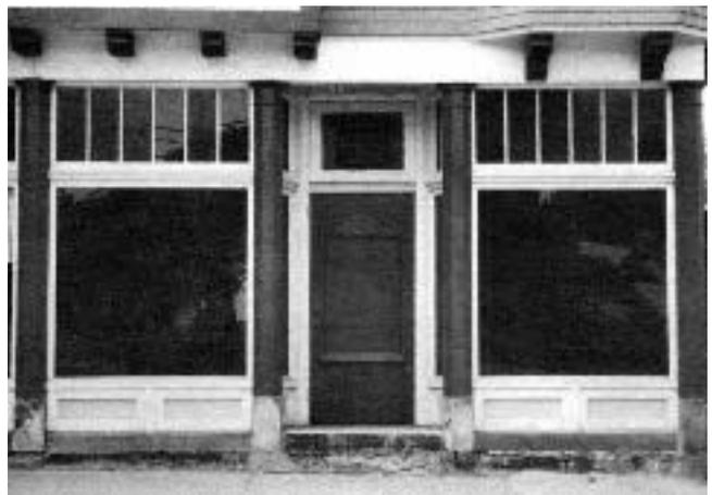
Figure 7. A "simulated storefront," (top), has a dark painted wall sitting behind the glass. It maintains the spacing of windows and entrances along the street (bottom), but makes the tenants feel more secure.
